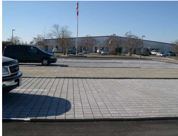
Figure 1. Permeable pavement parking lot in Kinston
