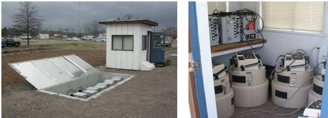
**Figure 4. Monitoring vault and shed (left) with detail of sampling equipment (right)**
