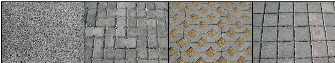
Figure 2. Permeable pavement sections consisting of (from left to right) porous concrete, Octabrick concrete pavers, concrete grid pavers, and Rima concrete stone
